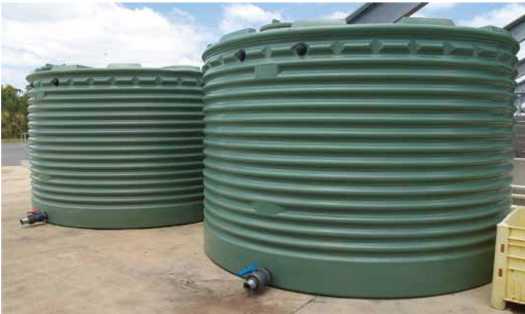
**Storage of high-strength waste for distillation at the Yalumba Oxford Landing Winery. These tanks are conveniently located between the marc bays and grape receive area, ensuring ease of access for tankers and ease of access for marc bay drainage, fermenter sludges and spills in the crusher pit.**
