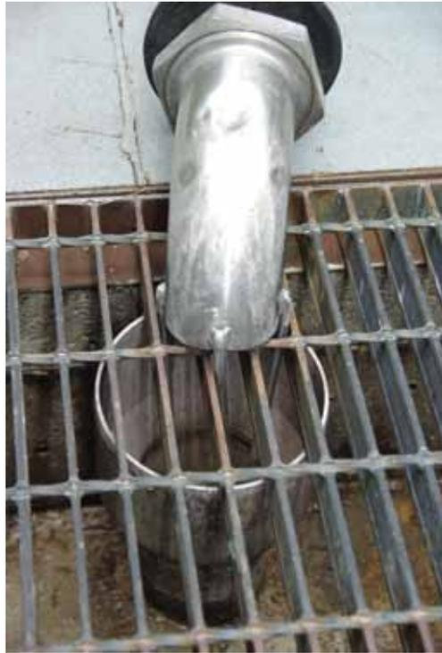
**Piped system for cellar wastewater within the cellar drains at the Yalumba Oxford Landing Winery.**
