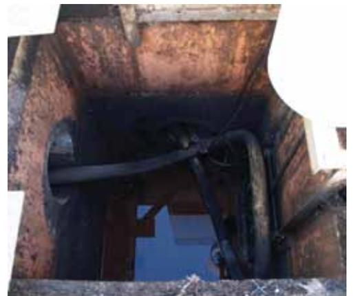
**Stormwater diversion sump at the Wolf Blass Winery, with the diversion to stormwater shown at the left side of the sump.** Photo courtesy of Rohan Wighton, Treasury Wine Estates.
