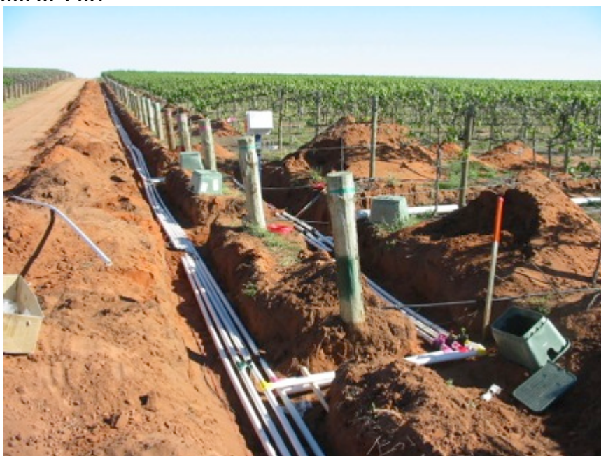
Figure 2 Installation of the irrigation controller, five new submains and pulse flowmeters.
