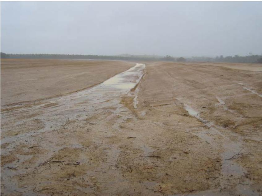
Figure 6. 'U' shaped channel on a roaded catchment.
